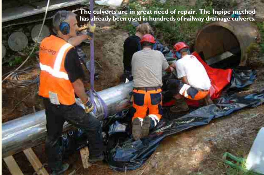
The Inpipe method works for most types of pipe and culvert, and manages diameters of up to 1,200 millimetres.
