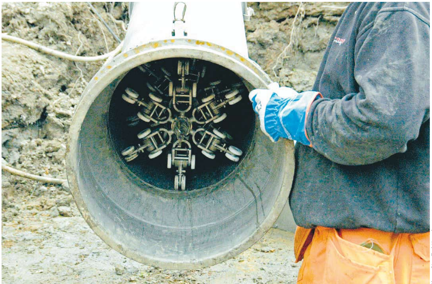
The tube of UV lamps is mounted at one end of the fibreglass liner and pulled through the culvert at a speed determined by the diameter size. The rays activate the hardening process.
