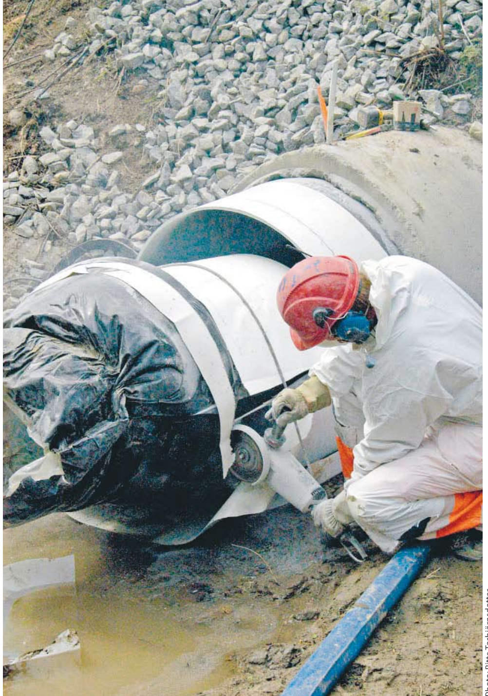
The Railcare Group cut off the excess fiberglass liner with a grinder. There is quite a bit of dust but a face mask is not deemed as absolutely necessary. The product is not regarded as hazardous.
