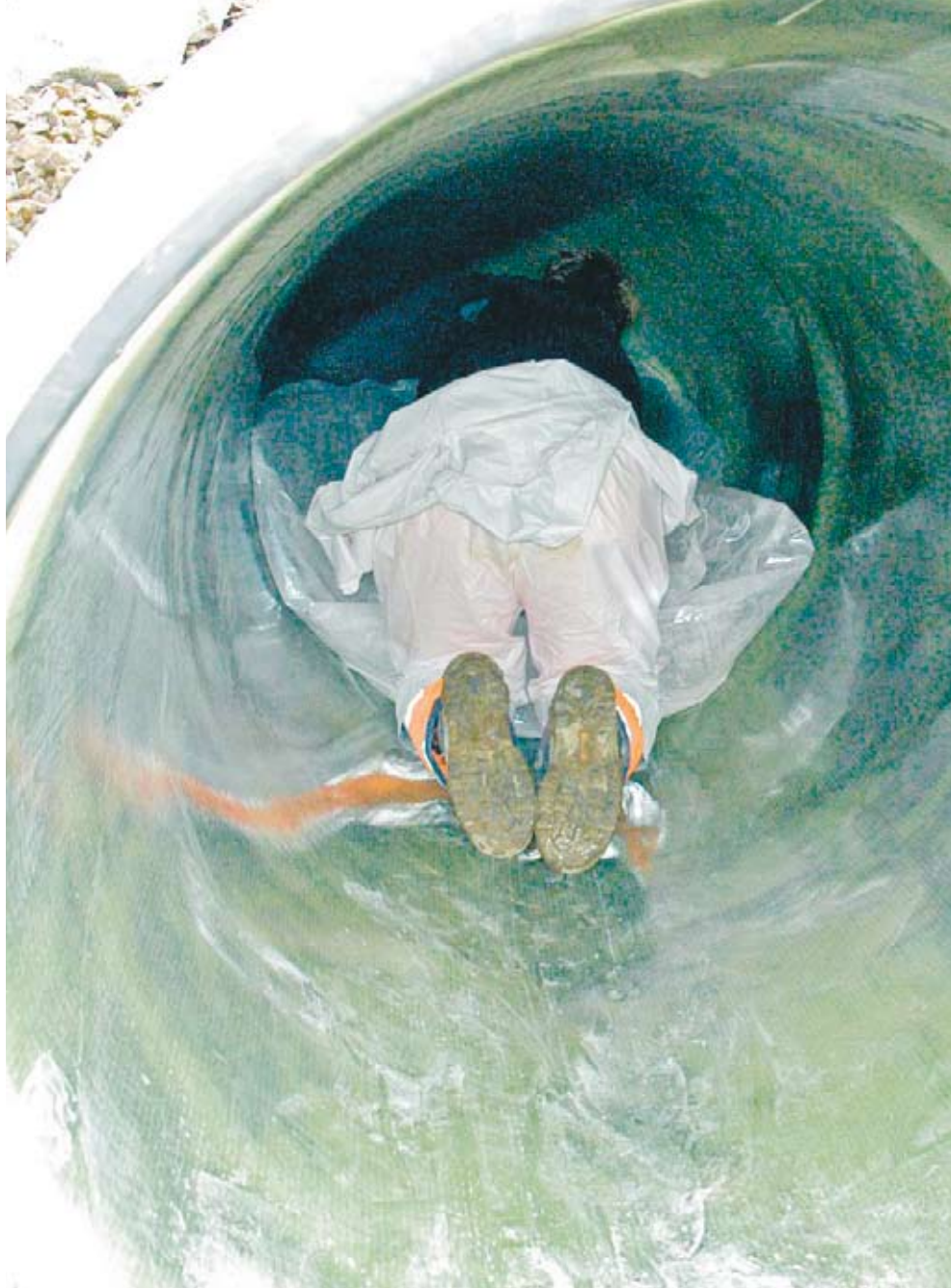
Kurt Boström creeps along the pipe liner to check it. Installation has as usual taken around eight hours, which is a significant timesaving compared to conventional digging.
