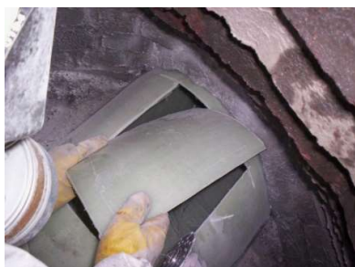
Figure 2, Suggestion for the socket for 3-point bend Figure 3, the overlap of fabrics in the finished liner
